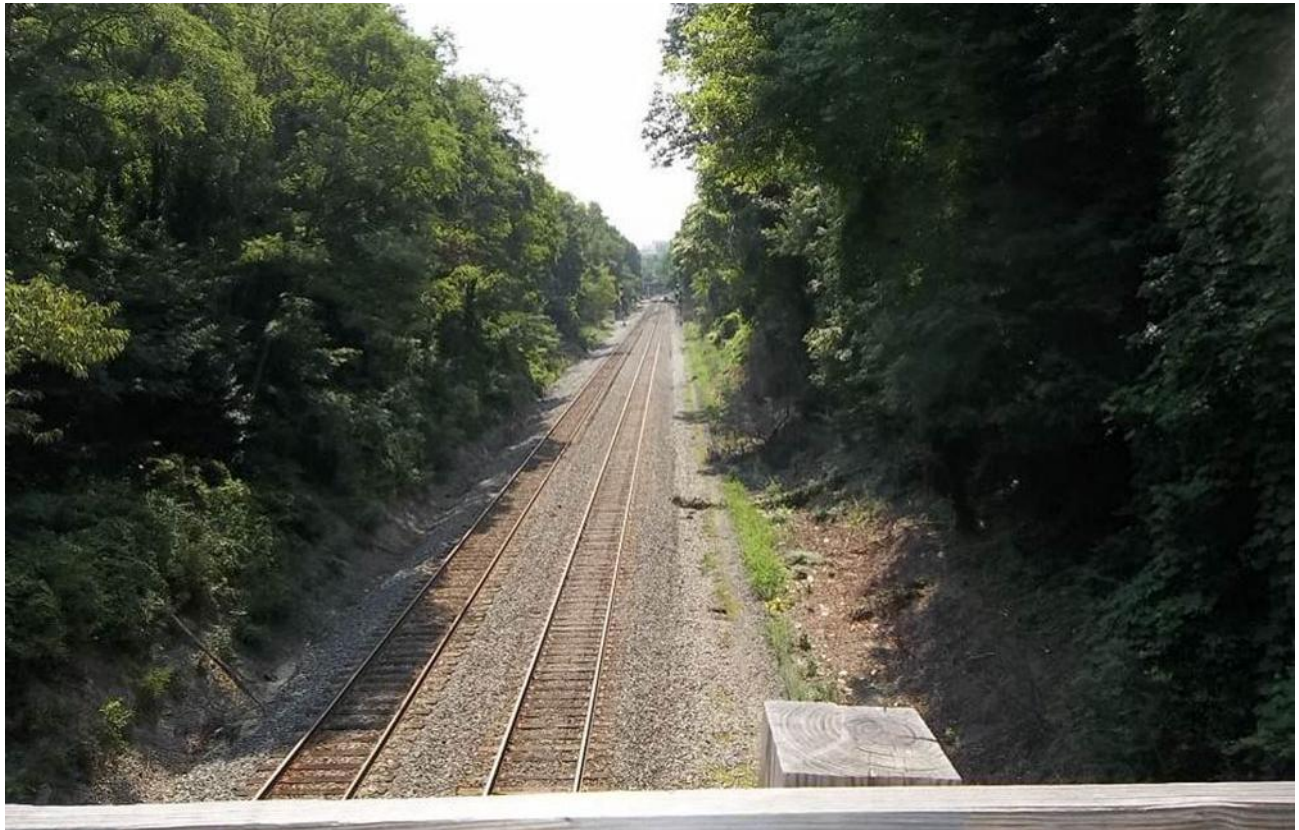
Figure 37. View Looking North from Talbot Avenue Bridge along Metropolitan Branch
