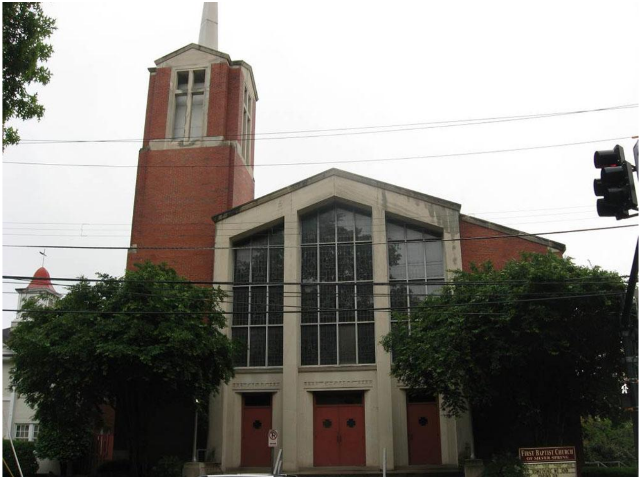
Figure 50. First Baptist Church of Silver Spring, South Elevation
