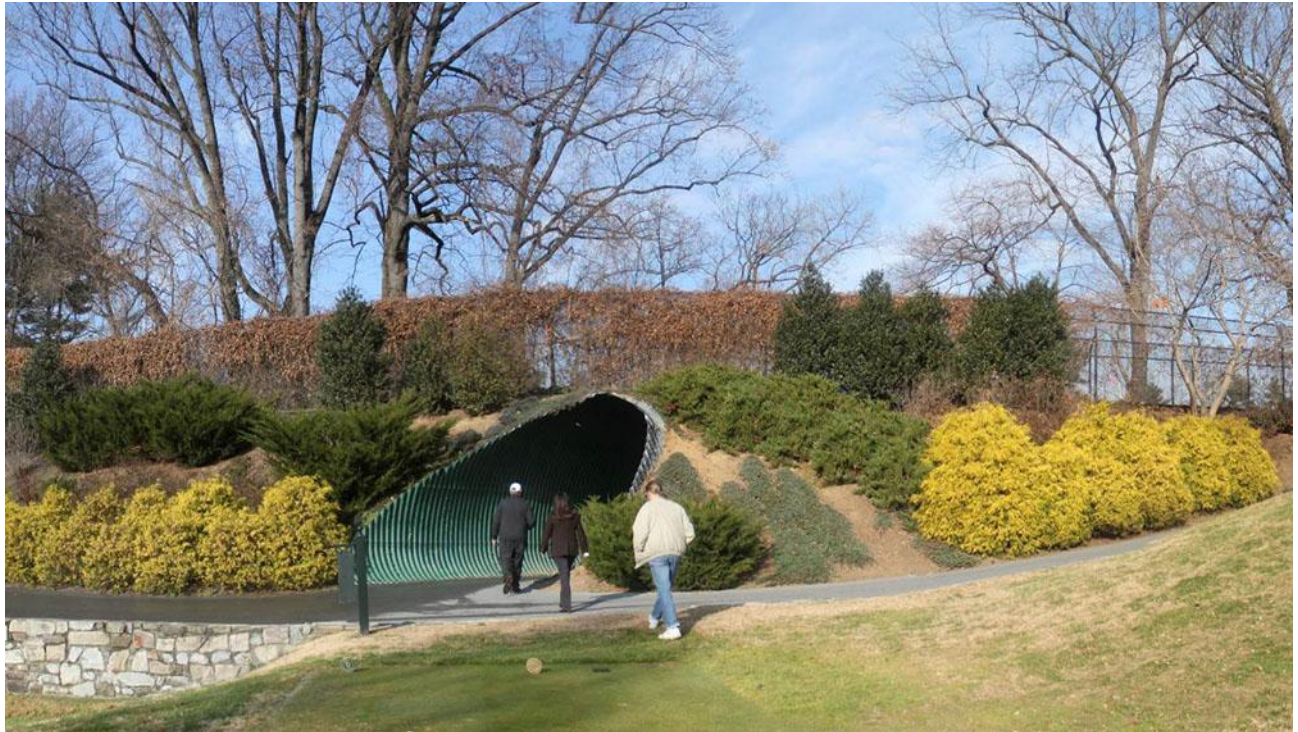
Figure 23. Existing East Underpass of the Georgetown Branch Right-of-Way, Looking Northwest
