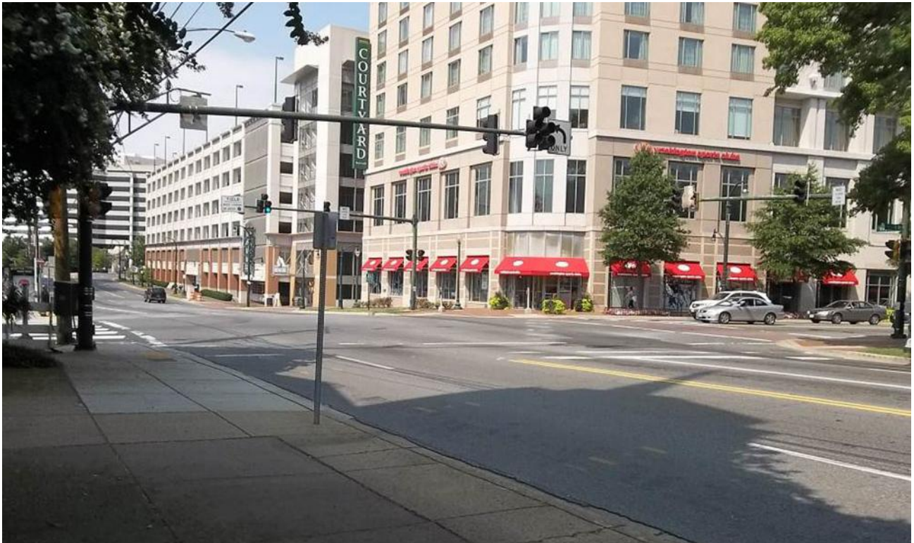
Figure 52. Looking Northwest from First Baptist Church of Silver Spring to Proposed Purple Line Alignment
