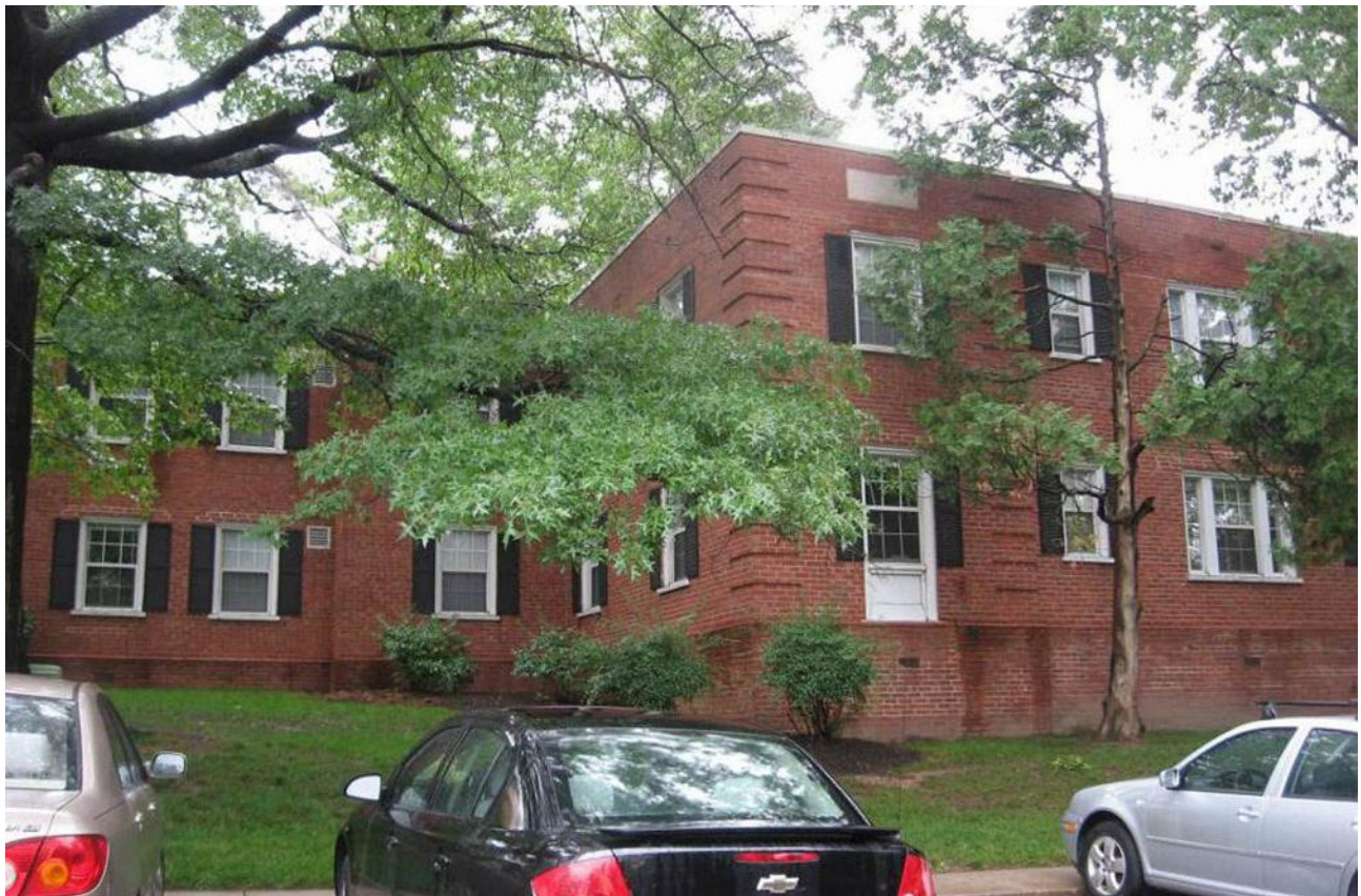
Figure 43. The Falkland Apartments
