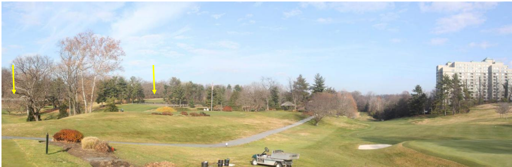
New parapet wall noted by yellow arrows. Note the modern apartment building within the viewshed to the right.
