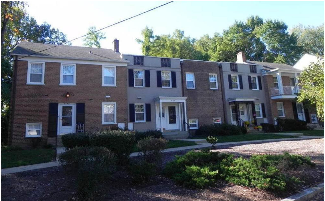
Figure 26. Preston Place Townhomes
