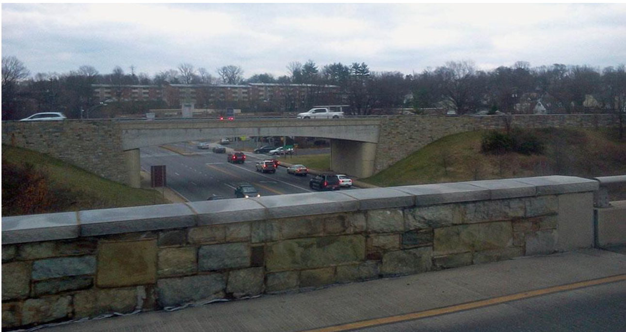
Figure 86. Detail of Existing Southbound Bridge Stonework, Looking Southeast
