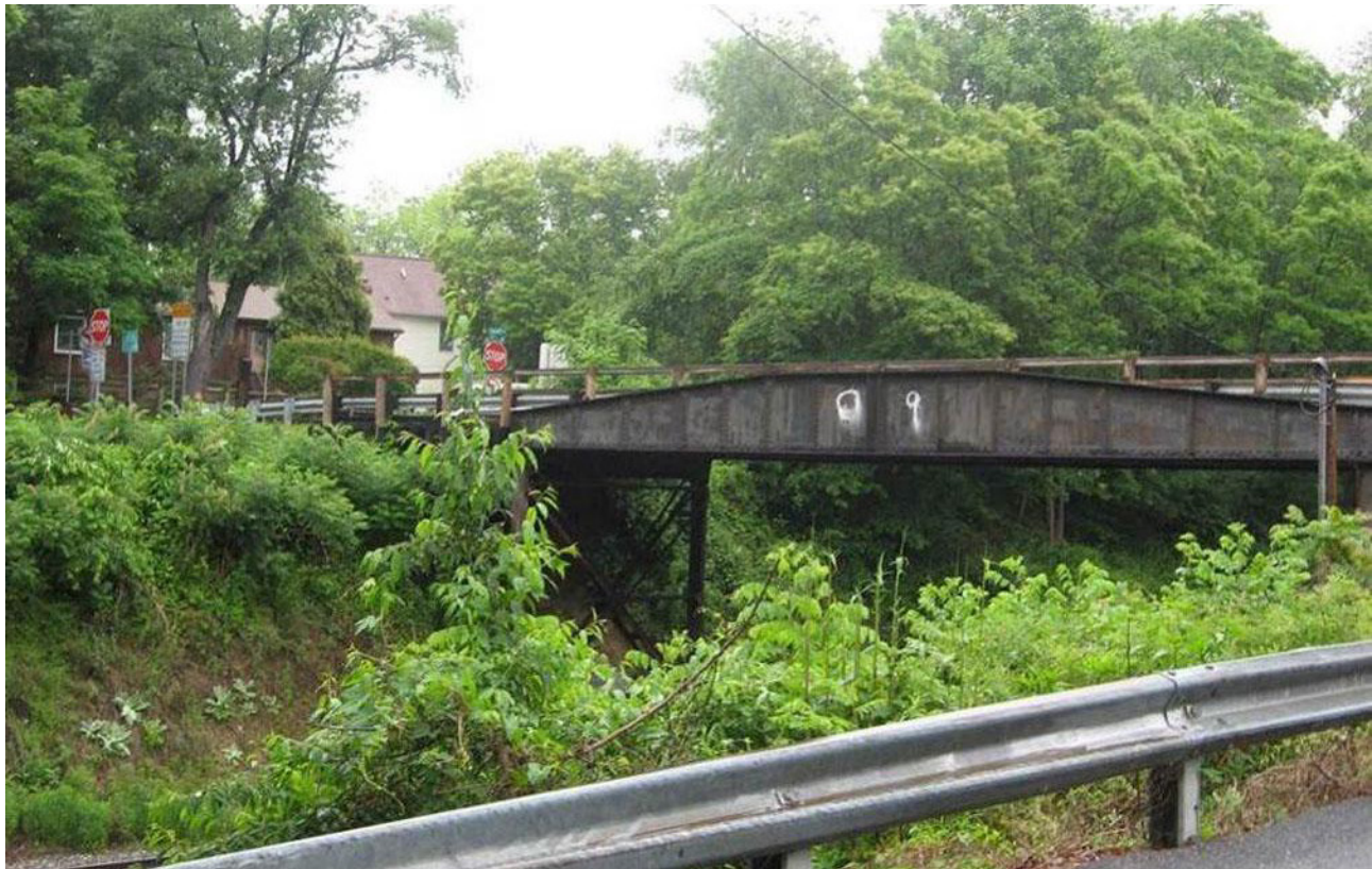
Figure 35. Talbot Avenue Bridge Spanning the Metropolitan Branch Railroad, North Elevation
