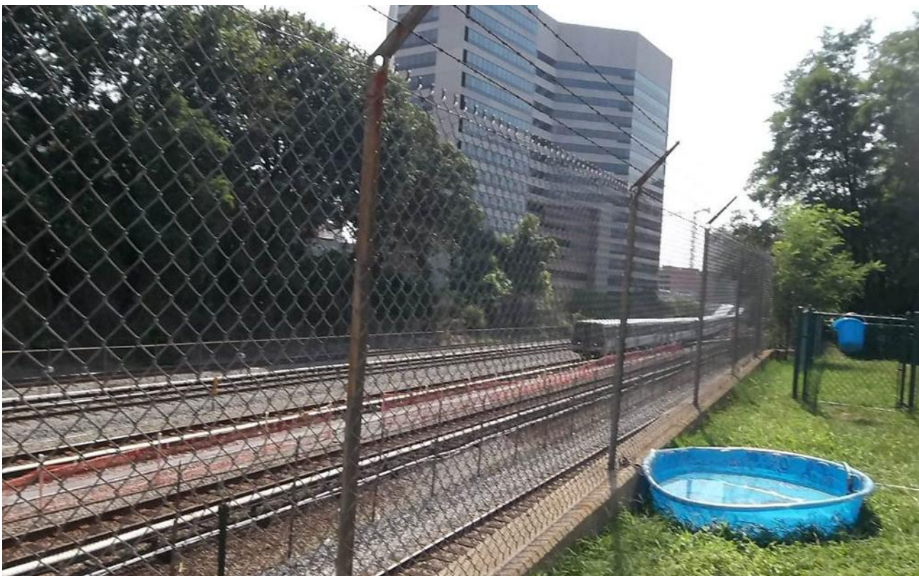
Figure 45. Metropolitan Branch Railroad adjacent to the Falkland Apartments
