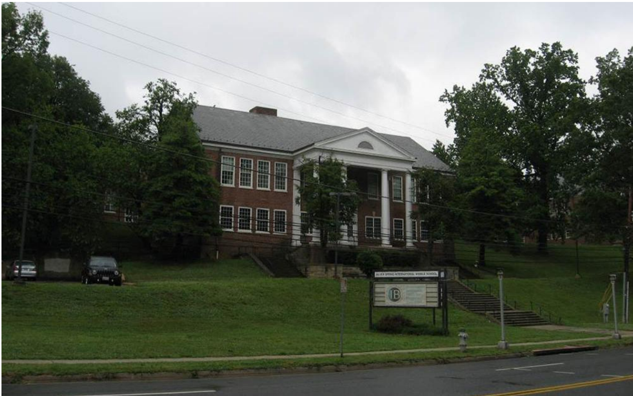
Figure 53. View Looking North from the Proposed Purple Line Alignment to the High School
