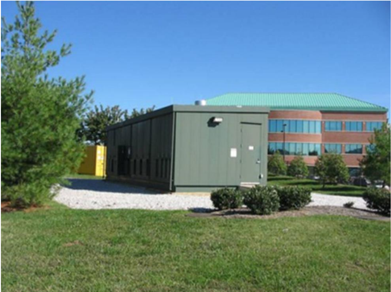
Figure 6. Traction Power Substation
